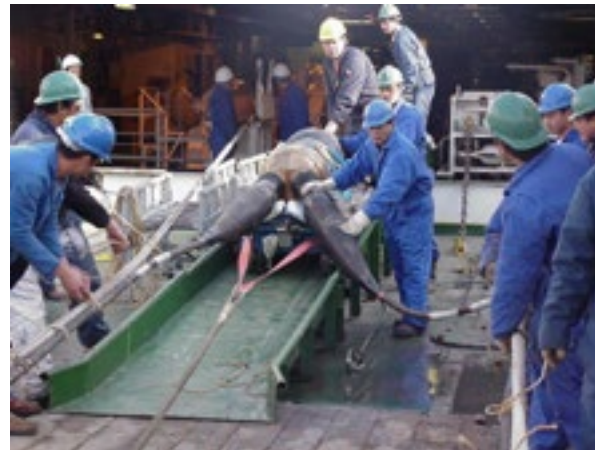
Figure 8 – Workers prepare for Cable laying
